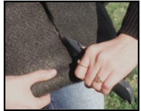
Cut Multi-Flow collector lines to the desired length using a utility knife.
